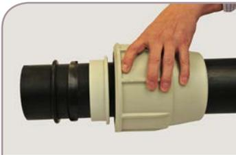
Draw the nut, collars, and O-ring over the end of the pipe to a distance of approx. 250mm (put the white split ring to one side for later use).
