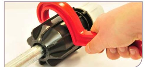
Tighten the black nut using a Plasson wrench or similar. Assemble the Metric PE joint as per the standard fitting instructions.
