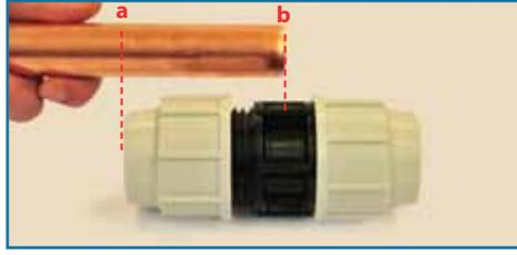
Place nut onto fitting leaving half the thread visible. Cut the copper pipe square and remove all burrs and sharp edges. Mark pipe at "a" when the pipe end reaches the centre of the body of the fitting, as shown by "b" above.
